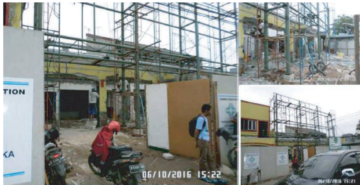
PT. Persada Medika - Building Assessment – Roof Garden RS. Jati Rahayu Bekasi 2016
